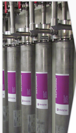
Biogas Upgrading Membrane Technology
